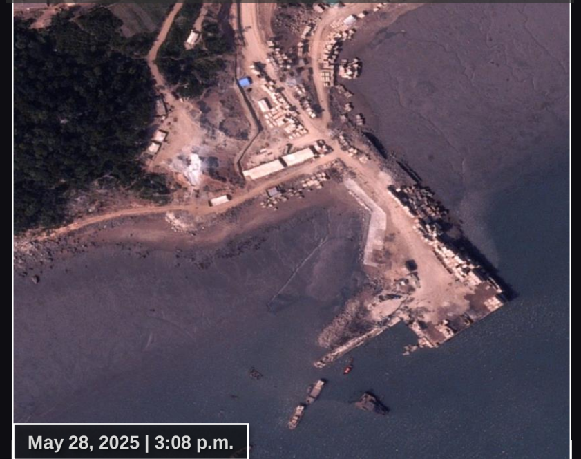
Sohae Satellite Launch Facility, North Korea
