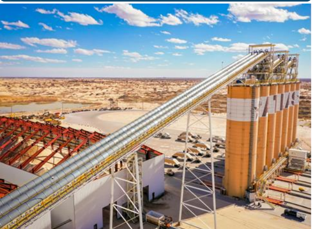
Atlas Conveyor Fed Silos at Kermit Facility
