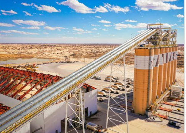
Atlas conveyor fed silos at Kermit Facility
