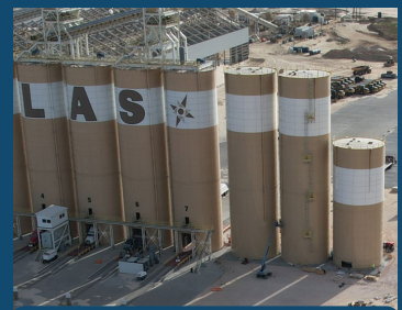
Silos currently going up
