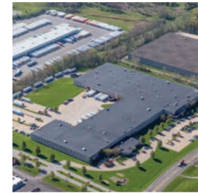
2100 International Parkway 274,464 square feet Canton, OH
