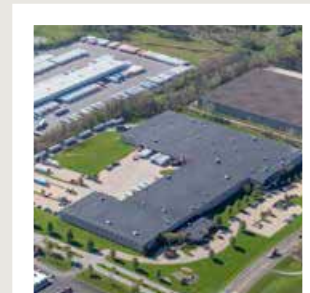
2100 International Parkway 274,464 square feet Canton, OH
