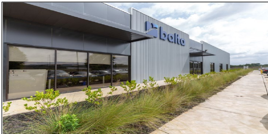
6739 New Calhoun Highway NE, Atlanta, GA
