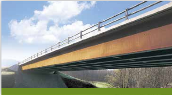
Steel bridges in the U.S.A. are increasingly using new high-performance steels (HPS 50W, HPS 70W, HPS 100W) produced by Cleveland-Cliffs with FINELINE® practices for improved toughness.
