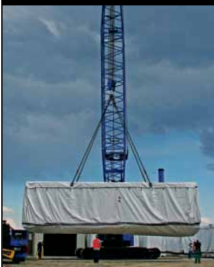
Receipt of condenser modules from Energy Northwest recycling project
