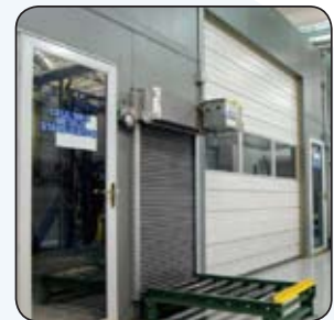
M&EC's facility expansion (SouthBay)
