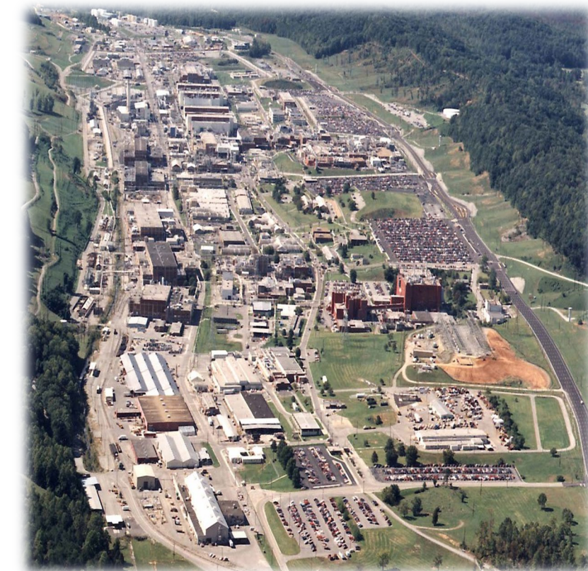
The Y-12 National Nuclear Security Administration facility in Oak Ridge, TN
