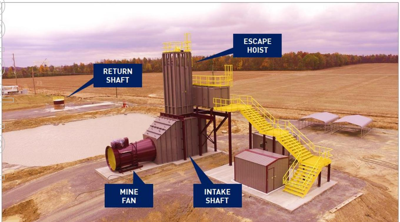
**Figure 1: Mine fan, intake shaft and return shaft mechanically complete and ready for commissioning**
