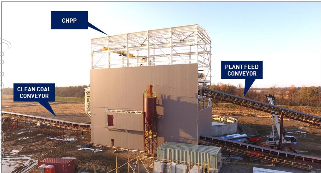
**Figure 4: Plant feed conveyor and clean coal conveyor complete at the CHPP**
