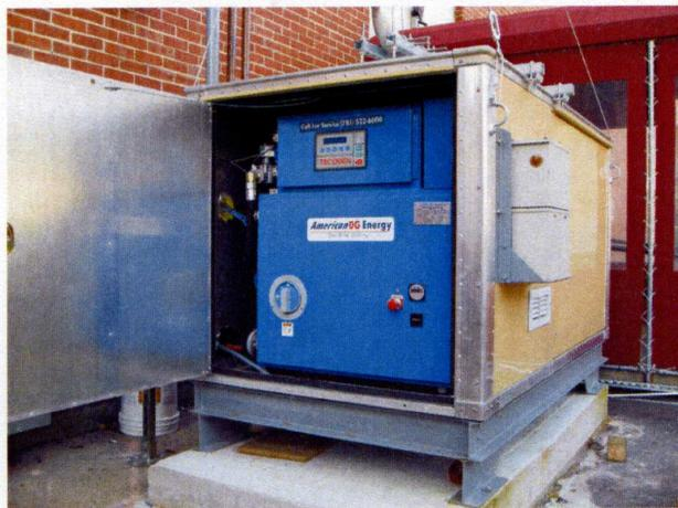
**A CHP system consists of an engine and a generator.**
