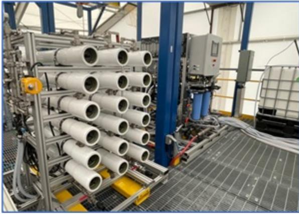
**The osmotically-assisted High Pressure Reverse Osmosis (HPRO) plant installed on the third storey of the Company's LiSTR DLE Plant. This unit acts as the link between the LiSTR DLE plant and the SiFT plant, and serves to concentrate the lithium chloride product so that it can be converted to lithium carbonate.**
