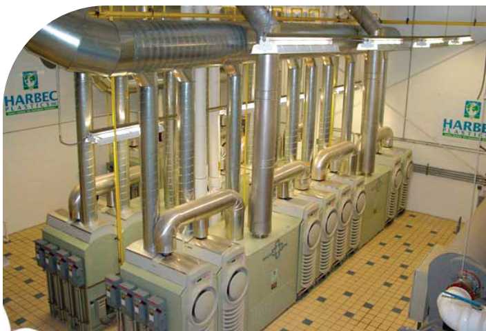
Harbec Plastics' original 25 C30 microturbines (left) were upgraded in 2015 with eight C65s (right) to expand capacity to support manufacturing needs while continuing to prioritize efficiency and sustainability.
