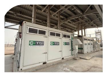
Two Capstone C600S microturbines power Basrah Gas Company's operations, utilizing waste flare gas to generate 1.2MW of clean energy. This efficient solution reduces emissions, eliminates diesel costs, and minimizes maintenance, enhancing operational efficiency and sustainability.
