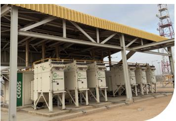
features two Capstone C600 Signature Series microturbines with a fuel gas skid, fire and gas detection systems and a customized high-efficiency filtration system.
