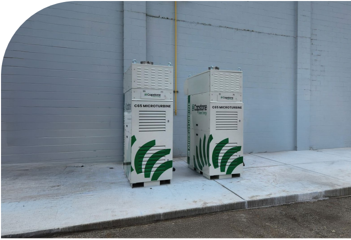
Two C65 ICHP microturbines installed at Strack & Van Til Food Market in Highland Indiana provide reliable power and to essential systems like refrigeration and check-out counters, ensuring uninterrupted critical functions.
