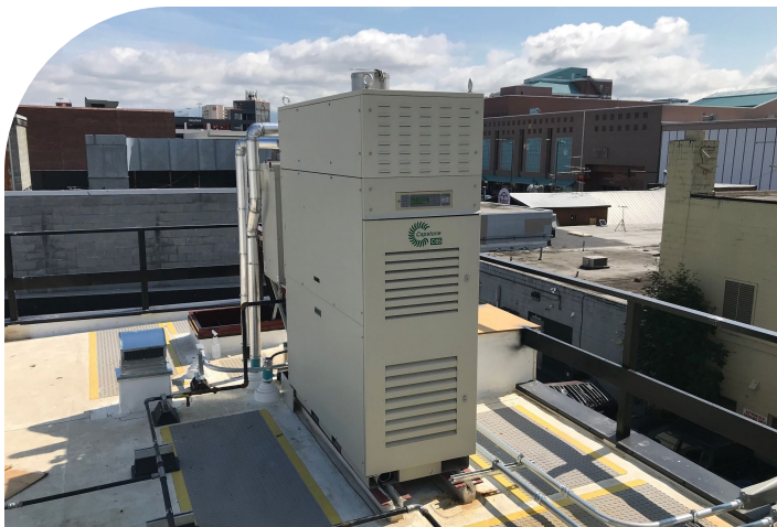
A Capstone C65 microturbine, situated on the rooftop of Whisky & Ramen in Anchorage, Alaska, delivers efficient power and heating with natural gas, achieving over 80% overall efficiency.
