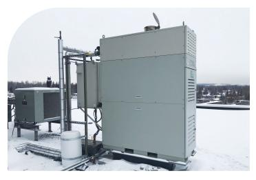
The Alutiiq Center in Anchorage features a Capstone C65 ICHP microturbine that significantly improves energy efficiency and reduces utility costs.
