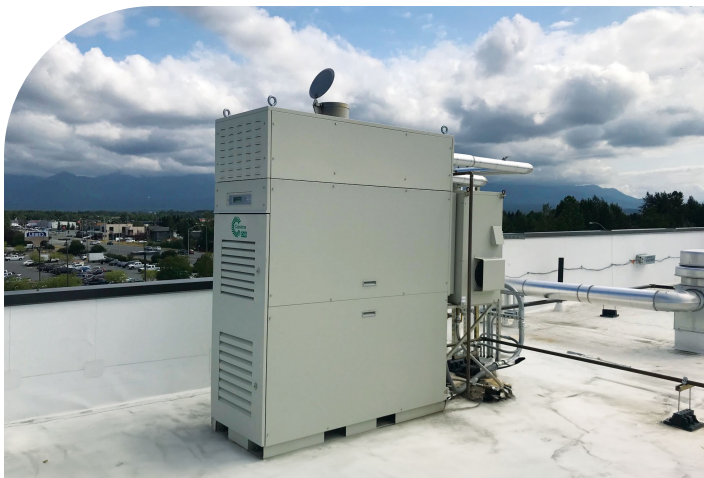
A C65 ICHP microturbines generates 65 kW of electrical power for Hyatt Place in Anchorage, Alaska.
