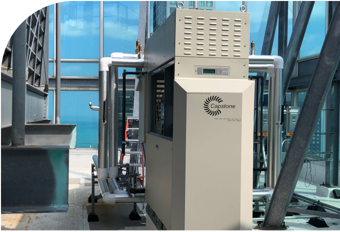
Two ICHP C65 microturbines fueled by natural gas provides Atwater Apartments, located in Chicago, reliable power while also reducing energy cost.
