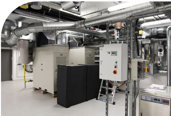
Two 65kW Capstone microturbines configured in a CHP application and a 3,000 MBTU/hr Heat Exchanger supply thermal power and electricity to the hospital.
