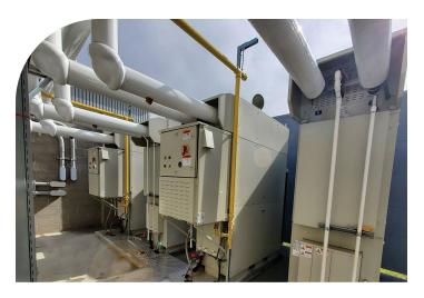
With the installation of four C65 ICHP Capstone microturbines, the Dryden Regional Health Centre has seen a reduction in annual electricity costs of over 50% while powering almost 100% of the hospital all winter and providing 100% of the heating for six months of the year.
