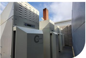
gas-fueled C65 microturbines, which replaced an old boiler. The microturbine array functions in grid connected operation, which allows the customer to operate in tandem with the utility while also alleviating strain on this remote section of the power grid.
