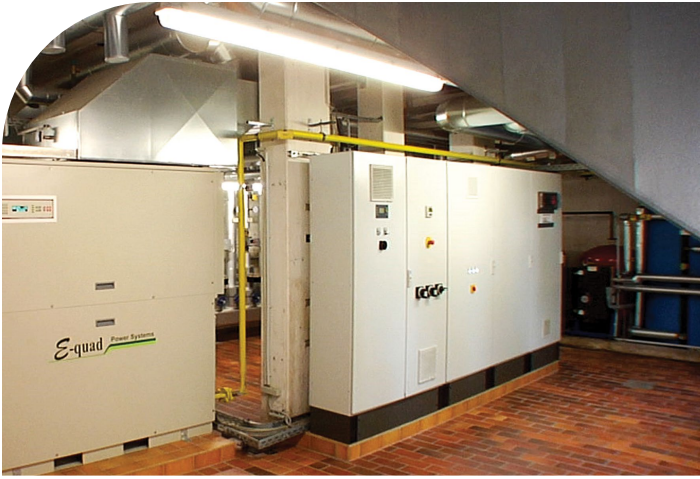
Two natural gas Capstone C65 microturbines make up the combined heat and power system at Catholic Hospital Koblenz in Augsburg, Germany.
