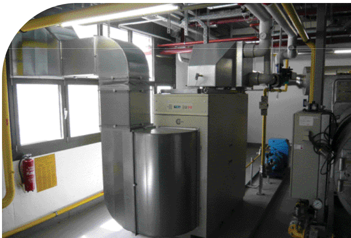
The Capstone C65 cogeneration system saves the hospital €22,500 annually in energy costs.
