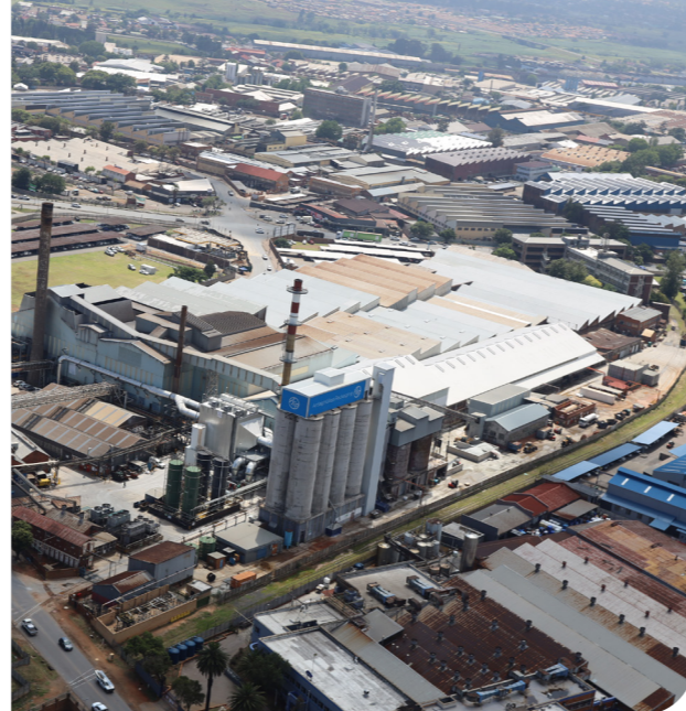
The installation of electrostatic precipitators (ESPs) across all our plants exemplifies our dedication to cleaner air.
