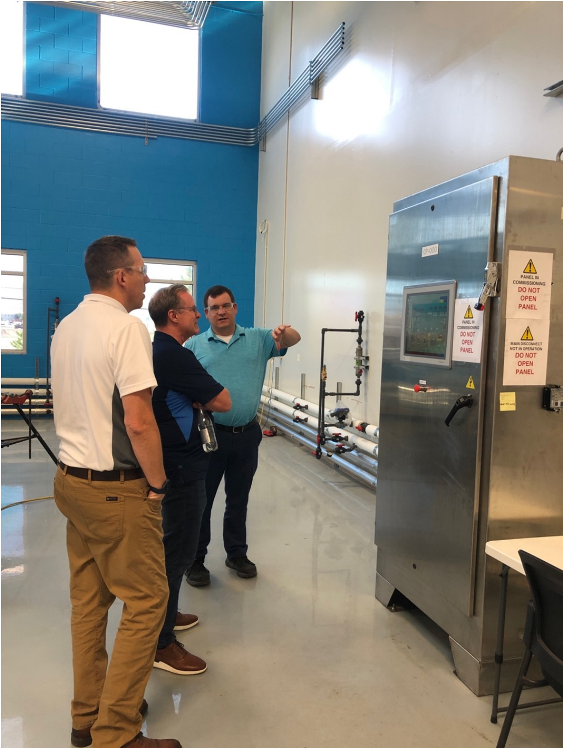
Jim Kenney, Director of Engineering, discusses the commissioning of the control panel for the Li AquaRefining pilot with CEO Steve Cotton and CFO Judd Merrill.
