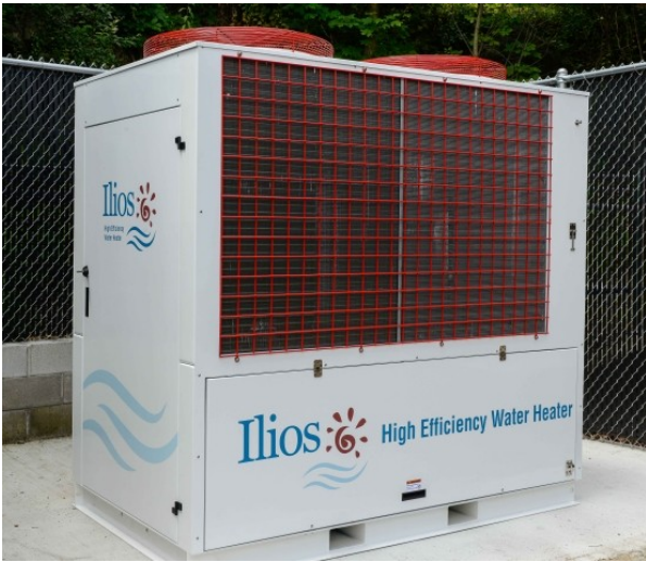
Typical packaged air-source gas engine-driven heat pump.
