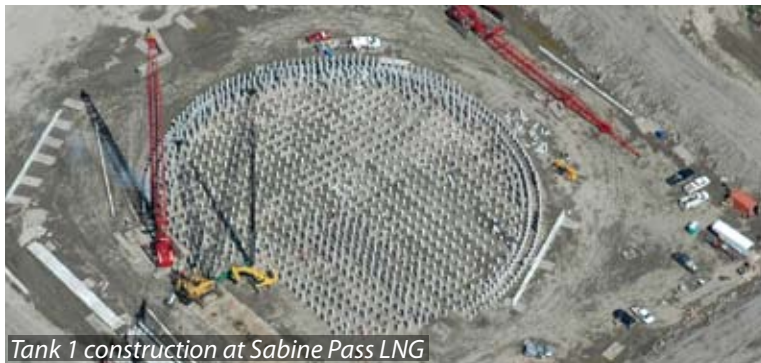
Pile driving at Sabine Pass LNG
