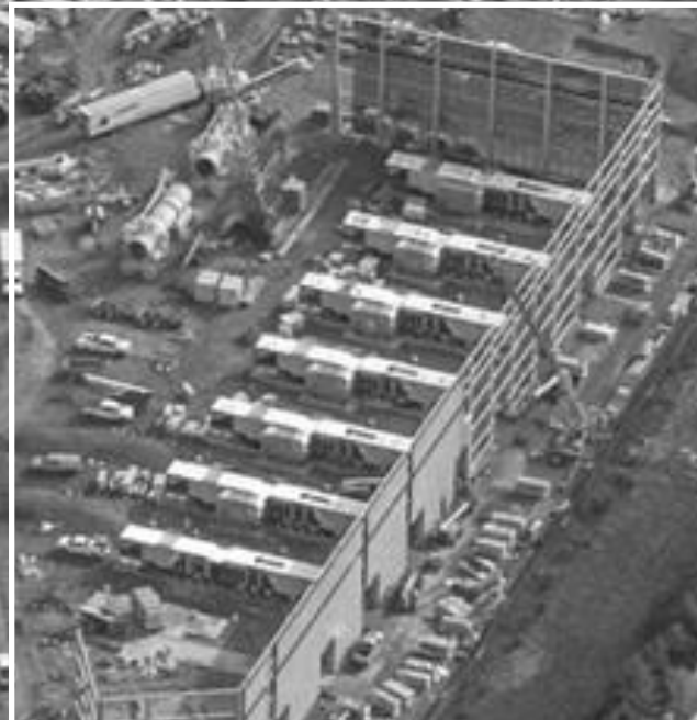
Kodiak Power Solutions Data Center Under Construction Solar SMT130 Turbines
