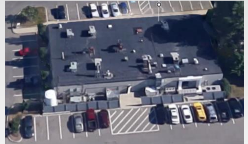
Odyssey's 10,000 sq. ft. wafer fabrication facility in Ithaca, NY
