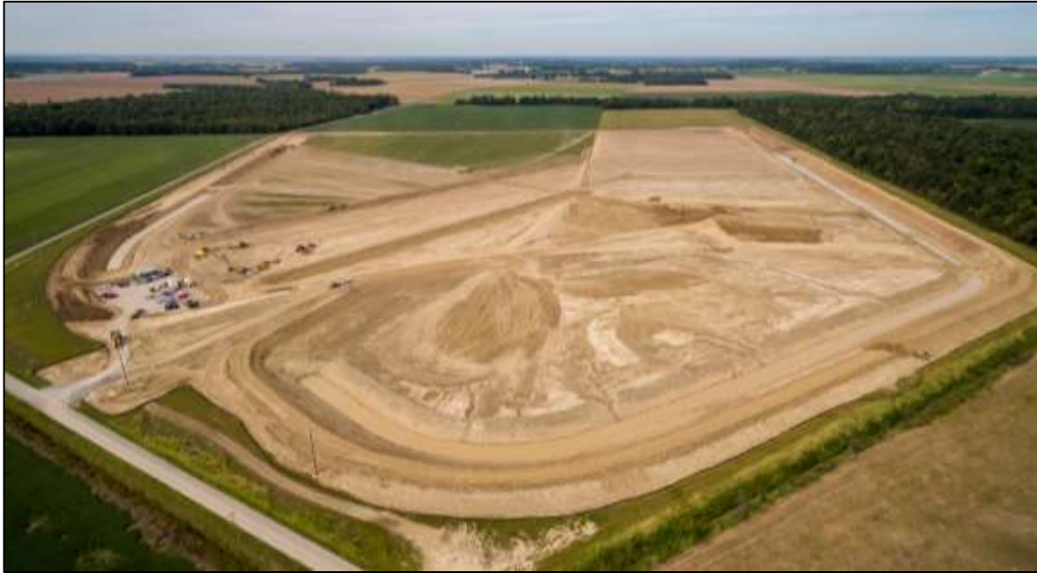
Site Excavation Continues at the Poplar Grove Mine
