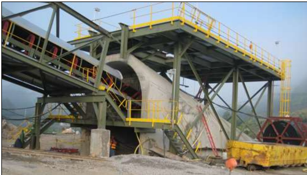
Example of a Slope Entry Similar to Poplar Grove Mine
