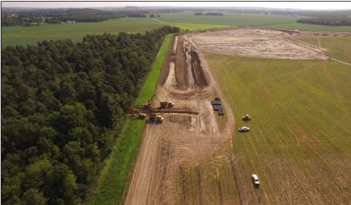
Construction of Levies Surrounding the Poplar Grove Mine
