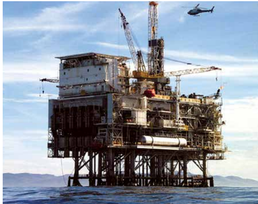
Forty six Capstone microturbines provide prime power to 27 offshore oil rigs in the Gulf of Mexico.
