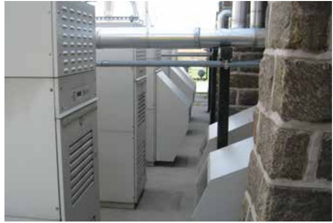
Capstone microturbines generate electricity and heating at Masonic Village, a 1,400-acre complex serving more than 2,000 residents since 1910.
