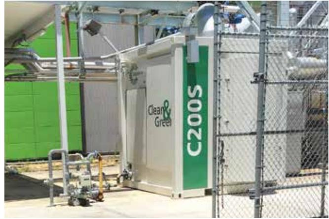
*A C200S microturbine is operated in a CCHP configuration, generating on-site electricity and recovering waste heat to power two 30-RT, hot-water-fired absorption chillers that base load the plant's heating, ventilation and air conditioning system.*
