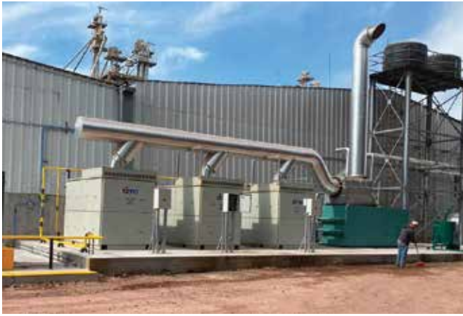
The microturbine-based CHP system at Forrajera 19 Hermanos was able to decrease their electricity bill by 93% and save more than $700,000 pesos ($32,200 USD).
