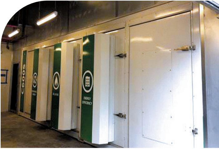
A 600 kW Capstone natural-gas-burning microturbine paired with absorption chiller and heat exchanger form the backbone of the microgrid for the office building and data center.
