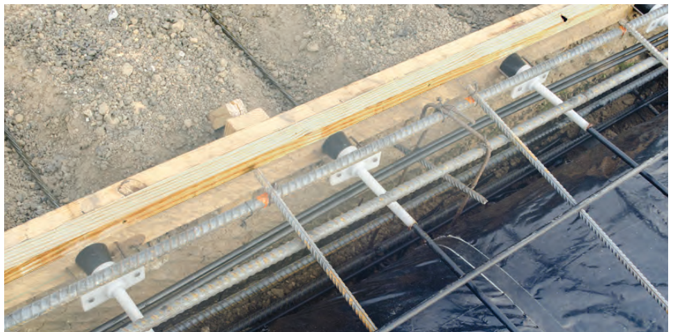
The Hayes Industries patented encapsulation anchors (seen in white) lead to better structural integrity and have recently been adopted into ACI and International Building Code
