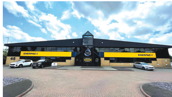
Site consolidation and investing in manufacturing capabilities make our Cramlington, UK facility a Center of Excellence for our torque and tension products.
