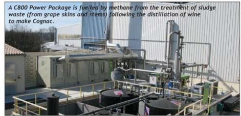
addition to the C800, the installation includes a Capstone-designed heat recovery module mounted inside the cabinet of the power package.
