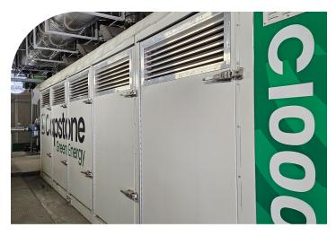
Two Capstone C1000S microturbines power Bardonecchia's highefficiency district heating network, delivering ultra-low emissions, 90% total system efficiency, and dependable operation in harsh alpine conditions.
