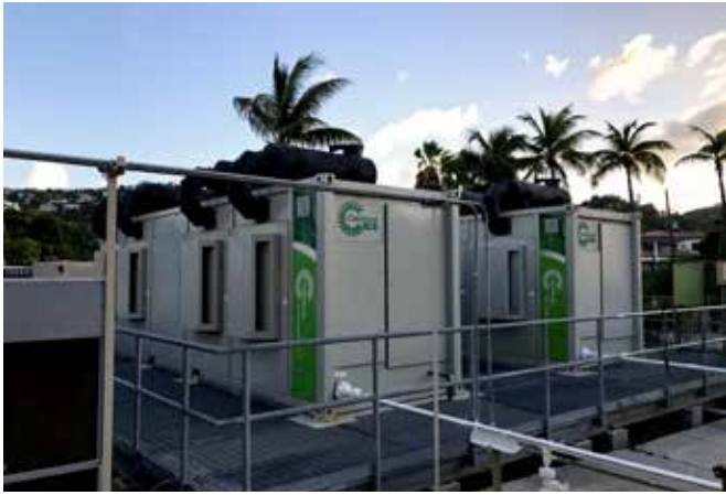
The on-site power plant at Margaritaville Vacation Club by Wyndham Resorts includes a 35,000-gallon propane storage tank that provides enough fuel to sustain on-site power generation for 14 consecutive days.
