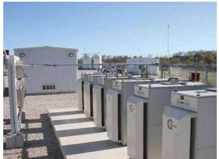
*Capstone microturbines, operating in the Eagle Ford and Marcellus shale plays, generate reliable and clean power.*
