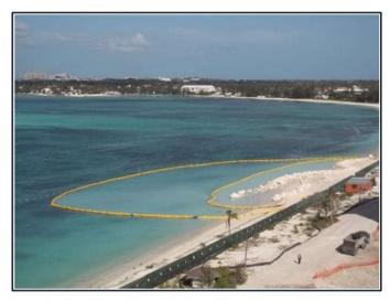
Photo 2. Example of a turbidity curtain utilized to contain turbidity. Photo from The Bahamas Weekly.
