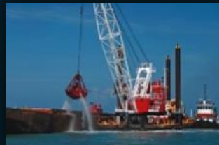
Dredging & Rock Dumping
