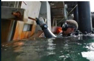
Dive Inspection Support
