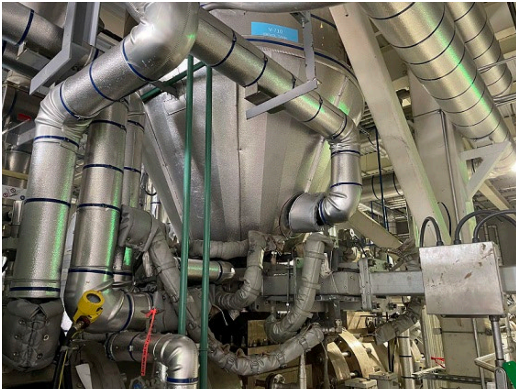
Figure 2: Insulated and Commissioned V-710 Devol Tank
