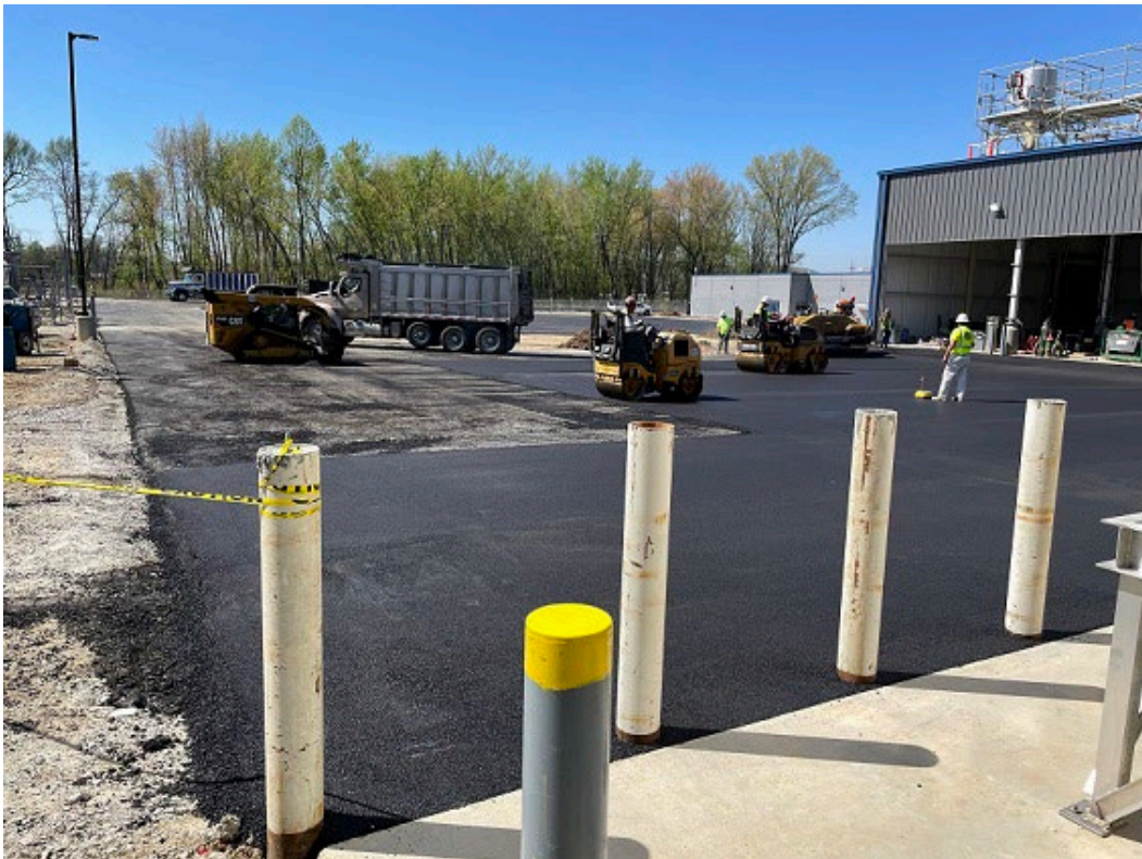
Figure 6: Commencement of Asphalt Paving
