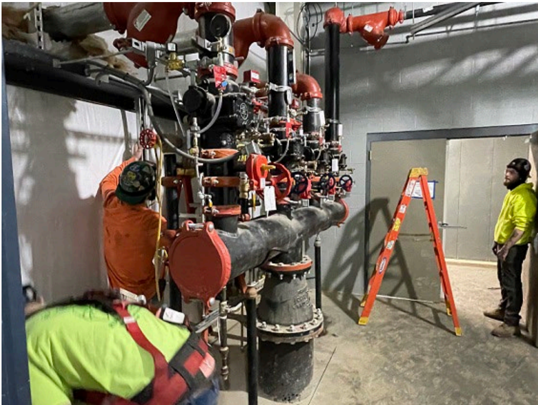
Figure 2: Installation of Fire Water Header near Extruder PK-720 in Building 610
