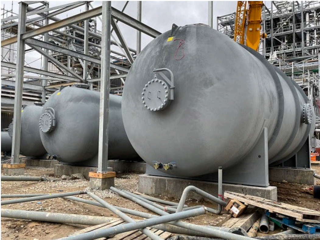
Figure 6: Installation of Knockout Drums
