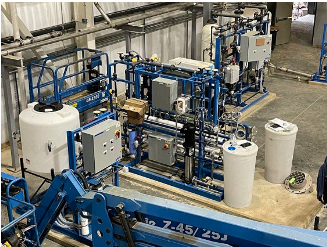
Figure 2: Installation of Reverse Osmosis System in Building 610
