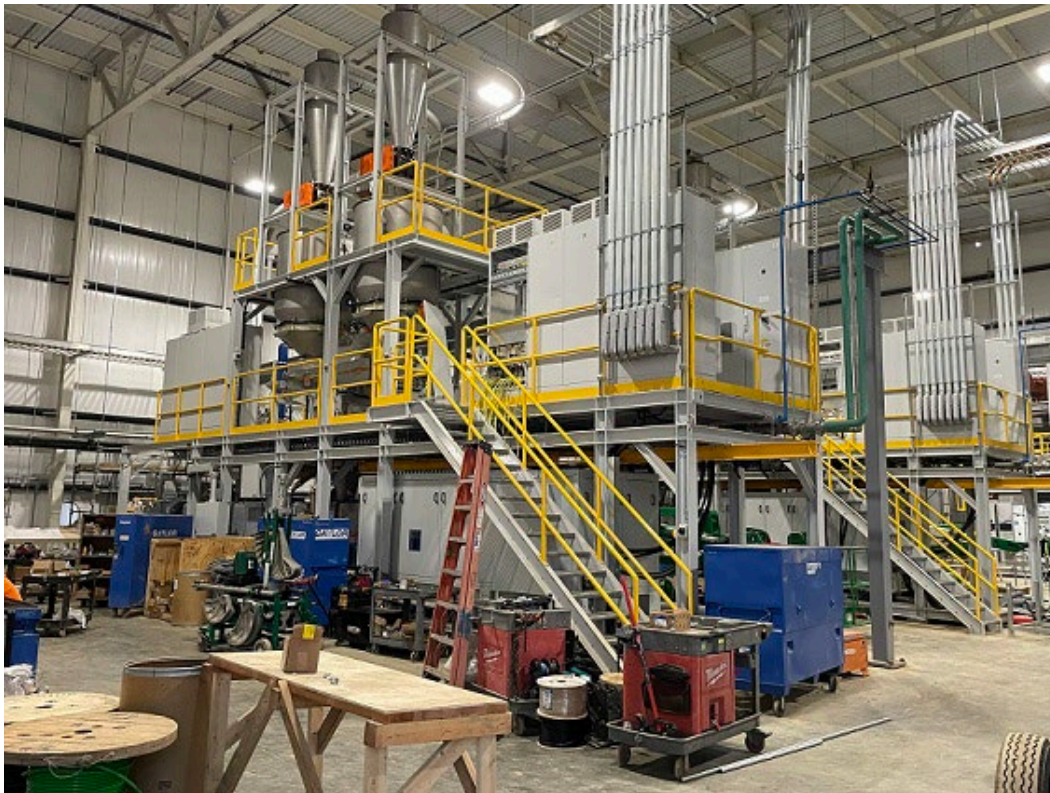
Figure 2: Installation of Reverse Osmosis System in Building 610
