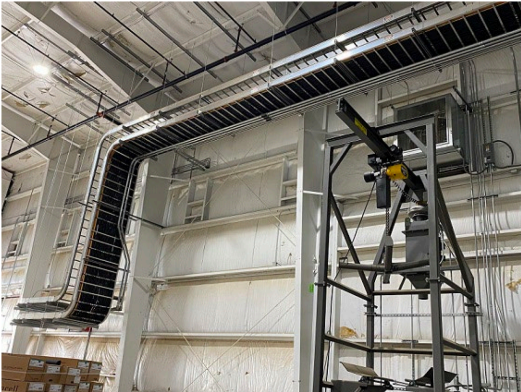
Figure 6: Pulling of Electrical Cable Through Cable Trays
